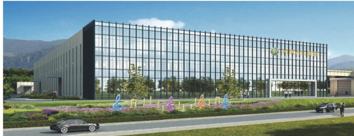
河南风尚电气配电柜建设项目 Henan Fengshang Electric Distribution Cabinet Project
