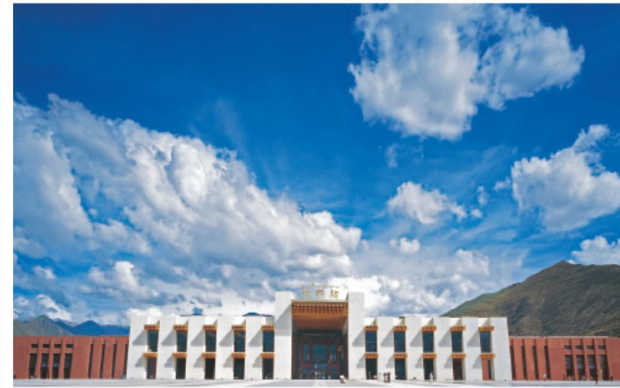
拉萨火车站 Lhasa Railway Station
