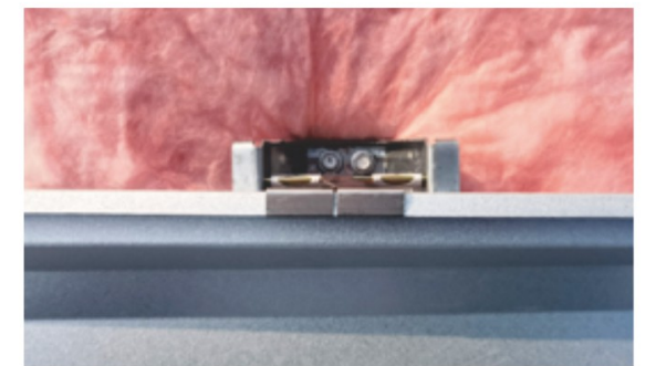
H75滑动支座及锁缝机 H75 Clip&Seaming Machine
