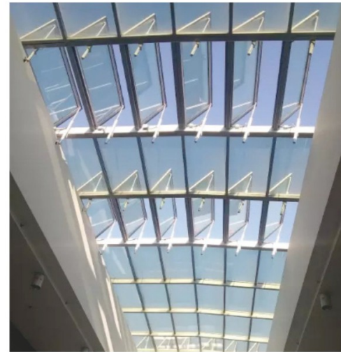
条形电动排烟玻璃天窗 Array-type Operable Glass Skylight and Smoke Vents
